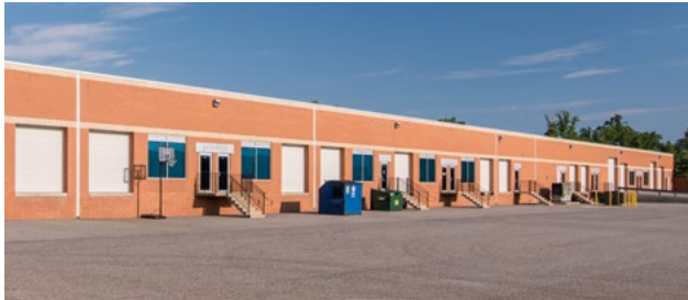
Flex/R&D dock and drive-in loading
