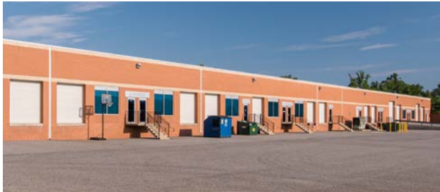
Flex/R&D dock and drive-in loading
