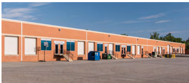
Flex/R&D dock and drive-in loading
