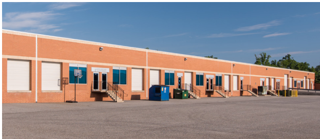
Flex/R&D dock and drive-in loading
