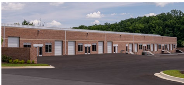
Top: Electric vehicle charging stations at 4961 Tesla Drive; Bottom: Drive-in loading with wide truck court
