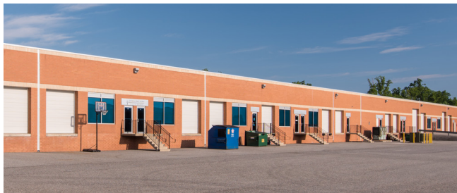
Flex/R&D dock and drive-in loading
