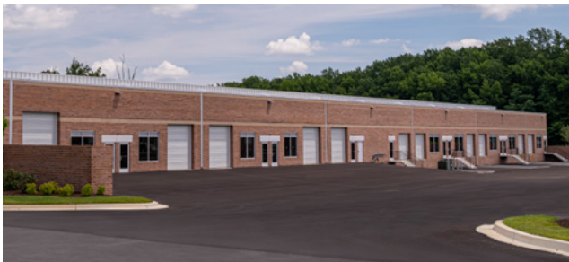
Top: Electric vehicle charging stations at 4961 Tesla Drive; Bottom: Drive-in loading with wide truck court
