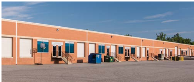
Flex/R&D dock and drive-in loading
