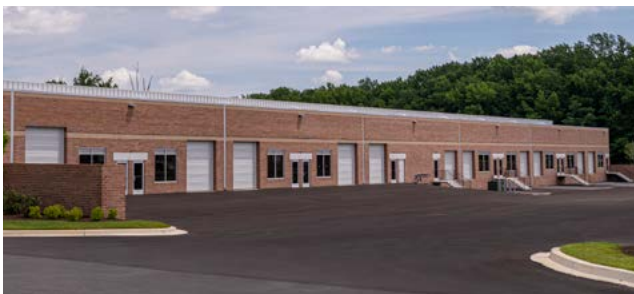
Top: Electric vehicle charging stations at 4961 Tesla Drive; Bottom: Drive-in loading with wide truck court
