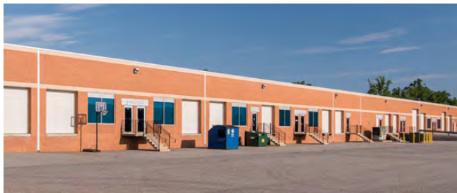
Flex/R&D dock and drive-in loading
