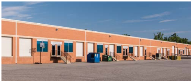
Flex/R&D dock and drive-in loading
