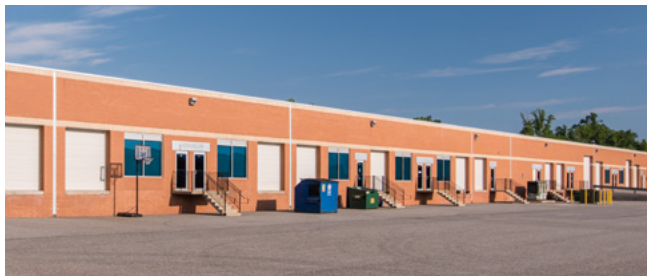
Flex/R&D dock and drive-in loading
