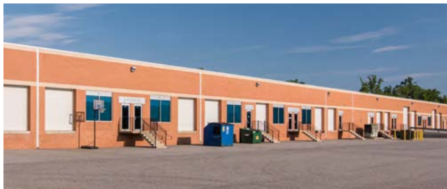
Flex/R&D dock and drive-in loading
