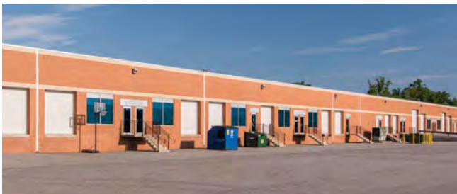
Flex/R&D dock and drive-in loading
