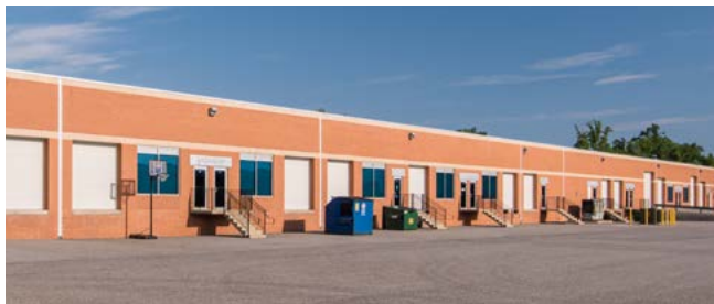
Flex/R&D dock and drive-in loading
